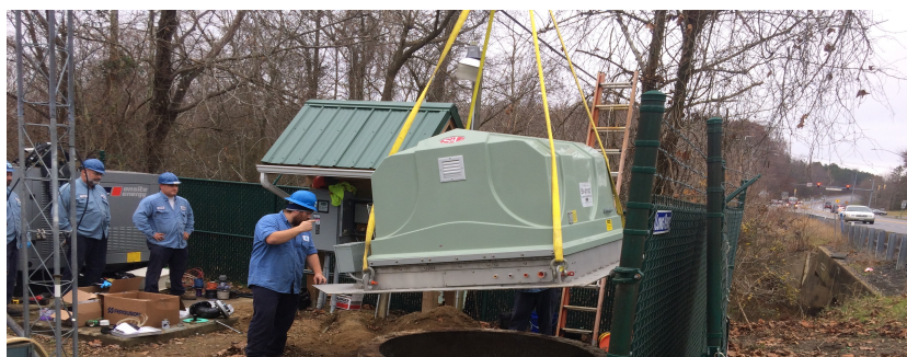
MetCom staff lowering a new packaged pump unit at the Glebe Run Wastewater Pumping Station
