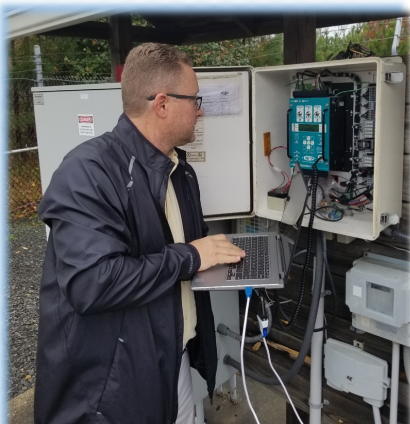
Programming SCADA Radios
