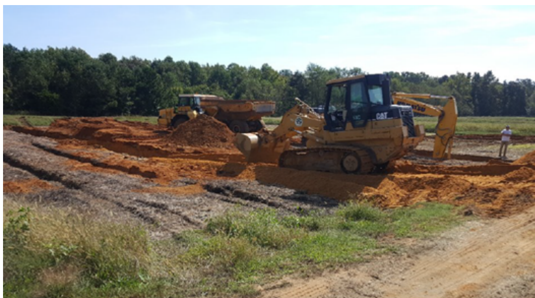
Installation of the sand trenches in the existing RIB facilities
