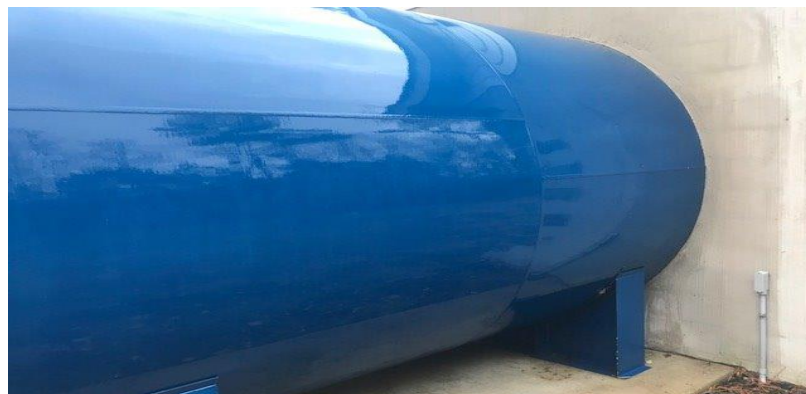
Forest Farm Repainted Water Pumping Station Hydro-Pneumatic Tank
