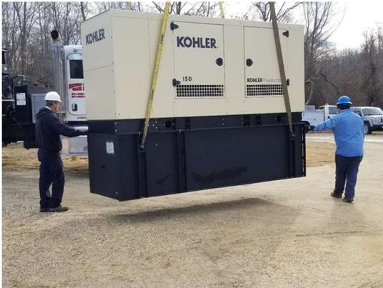
Staff installing a new emergency generator at the Wicomico Shores Wastewater Treatment Facility
