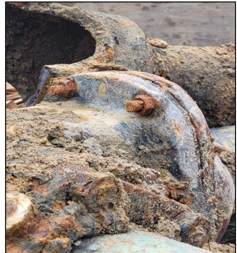
Pictured above are new stainless bolts installed on existing valves that have become corroded, increasing the likelihood of a failure.
