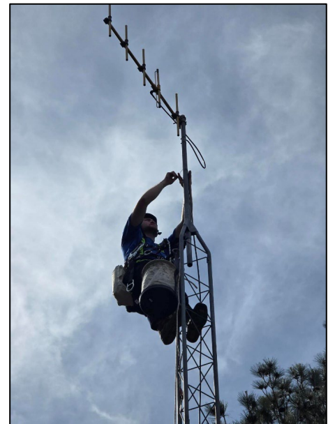
Staff performing SCADA equipment maintenance.
