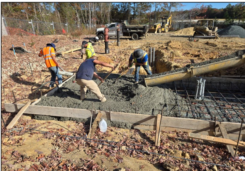
Bay Ridge Control Building Slab being poured.
