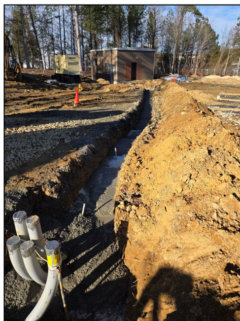
Electrical Conduit Installation At the Bay Ridge Well Site.
