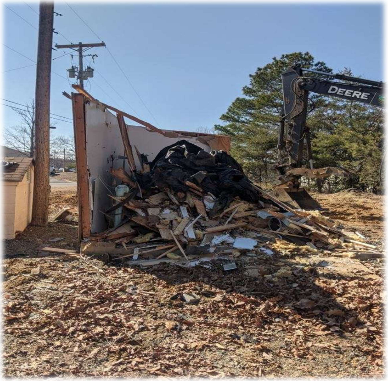
Demolition of Town Creek # 6 (Continued)
