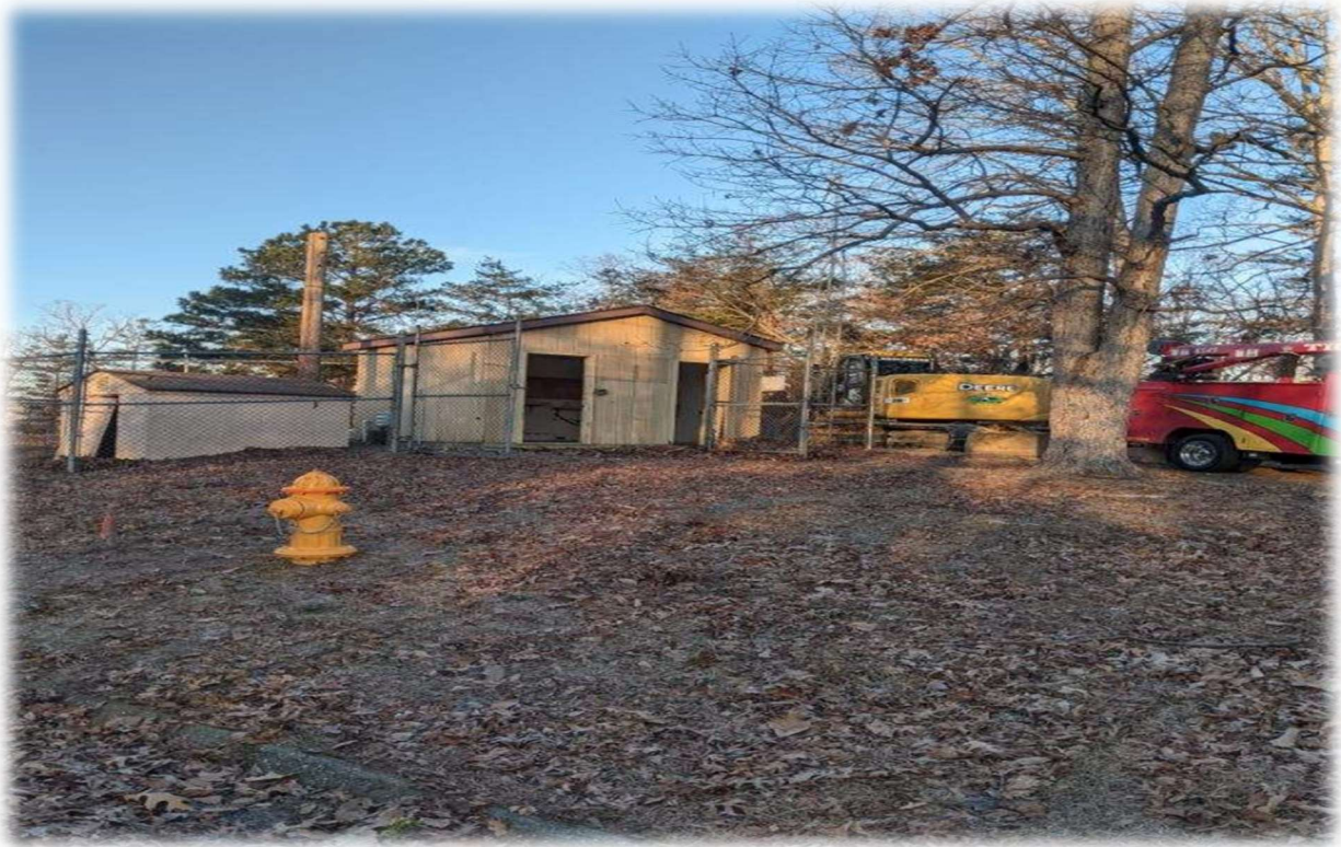
Demolition of Town Creek # 6 WPS
